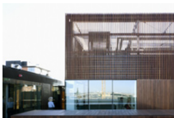
THE ROOF IS THE BUILDING'S 'FIFTH ELEVATION', A CONVIVIAL AMALGAM OF CAFÉ, GARDEN, KIDS' CENTRE AND OBSERVATORY. PHOTO BY DEAN KAUFMAN.
