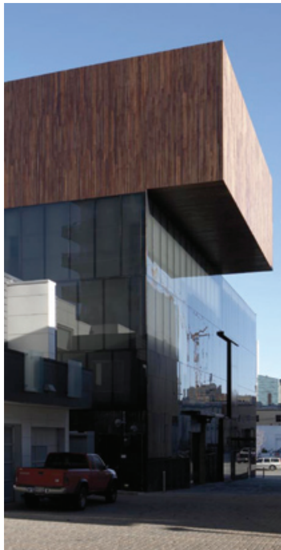
THE TAUT BOX IS WRAPPED IN BLACK GLASS WITH AN INNER LAYER OF LIGHT FILTERING INSULATION (MONOPAN). PHOTO BY ED REEVE.
