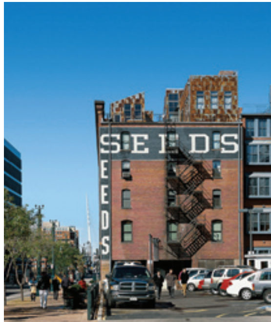
REMNANTS OF THE PAST MINGLE WITH MORE RECENT DEVELOPMENTS, EXEMPLIFIED BY THESE MODERN STRUCTURES SITTING ATOP AN OLD BRICK WAREHOUSE. PHOTO BY CAMERON WITTIG.
